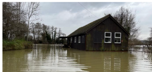
January 2024 where the water reached 80cms up the house (20cms higher than shown in this picture)
