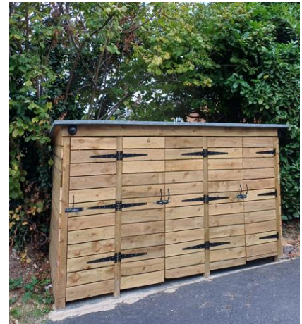
Bin store as built
