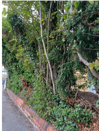
View along boundary with side of bin store just visible
