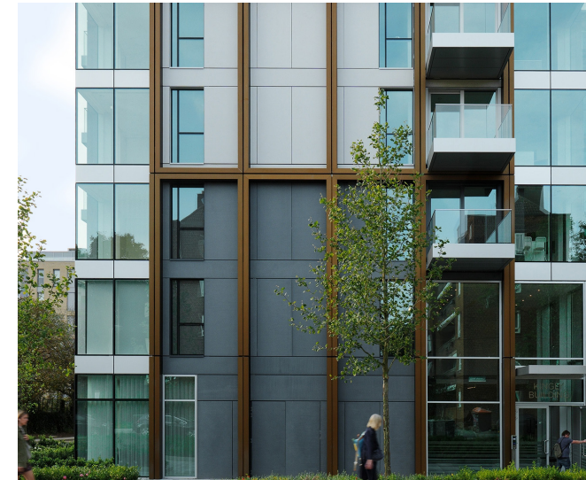
Fig. 2.24.3 - Metal & Glass Panels
