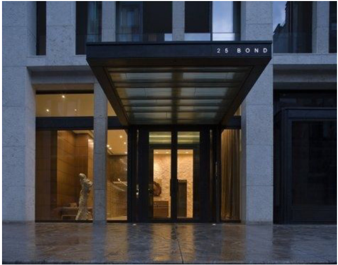
Fig. 2.18.2 - Weather protection at entrances
