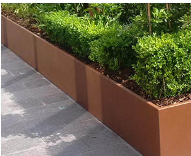
Fig. 3.6.5 - Raised Metal Edge To Planting
