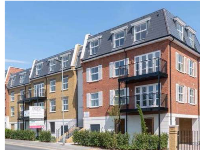
Elmwood Gate, Oldfield Road, Maidenhead
