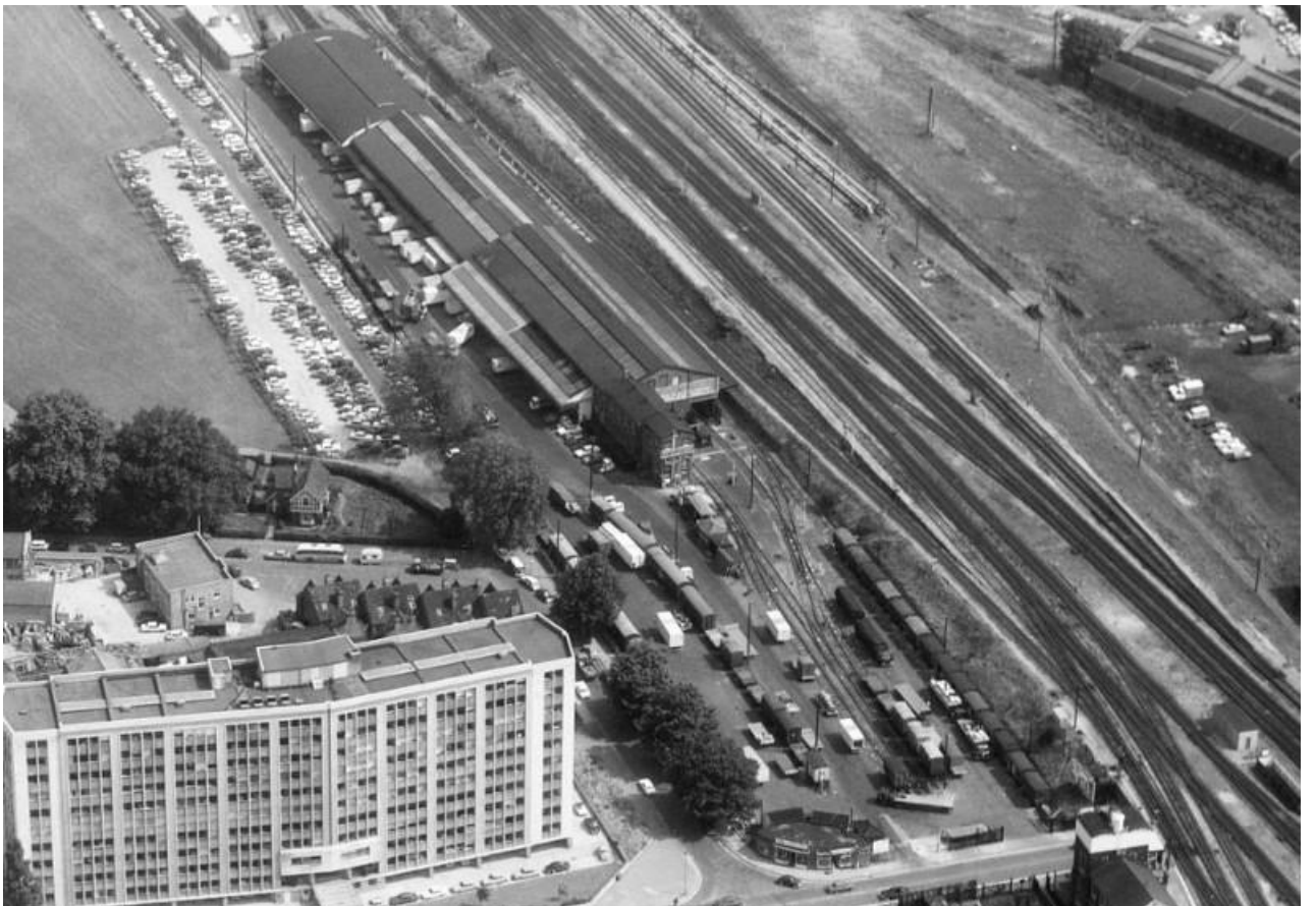
Figure 2.15 1962 air photo with car park along southern edge of The King's Meadow in front of the goods shed. Reading Bridge House in foreground. Source: Aerofilms EAW098027.
