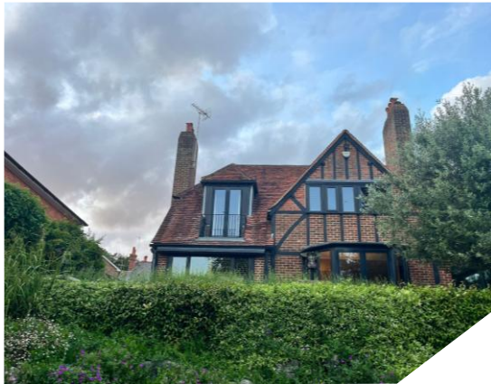
15. 29/05/2025, surveyor position, south-western aspect of B1.
