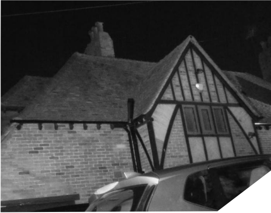
10. 29/05/2025, darkest point of survey, north-eastern aspect of B1.
