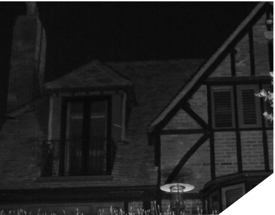
16. 29/05/2025, darkest point of survey, south-western aspect of B1.
