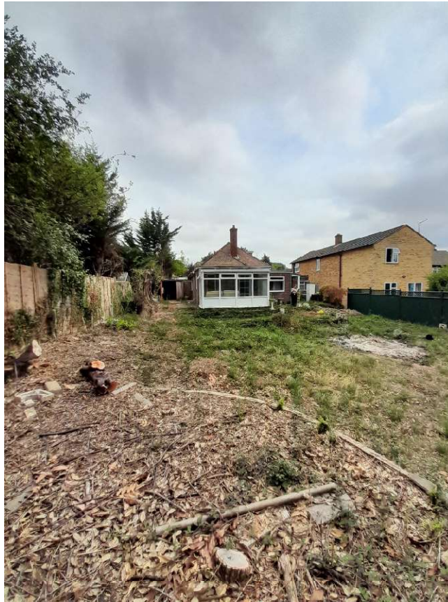
View of rear elevation looking northeast
