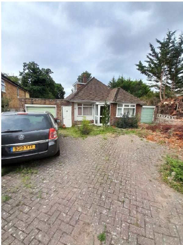
View of front elevation looking southwest
