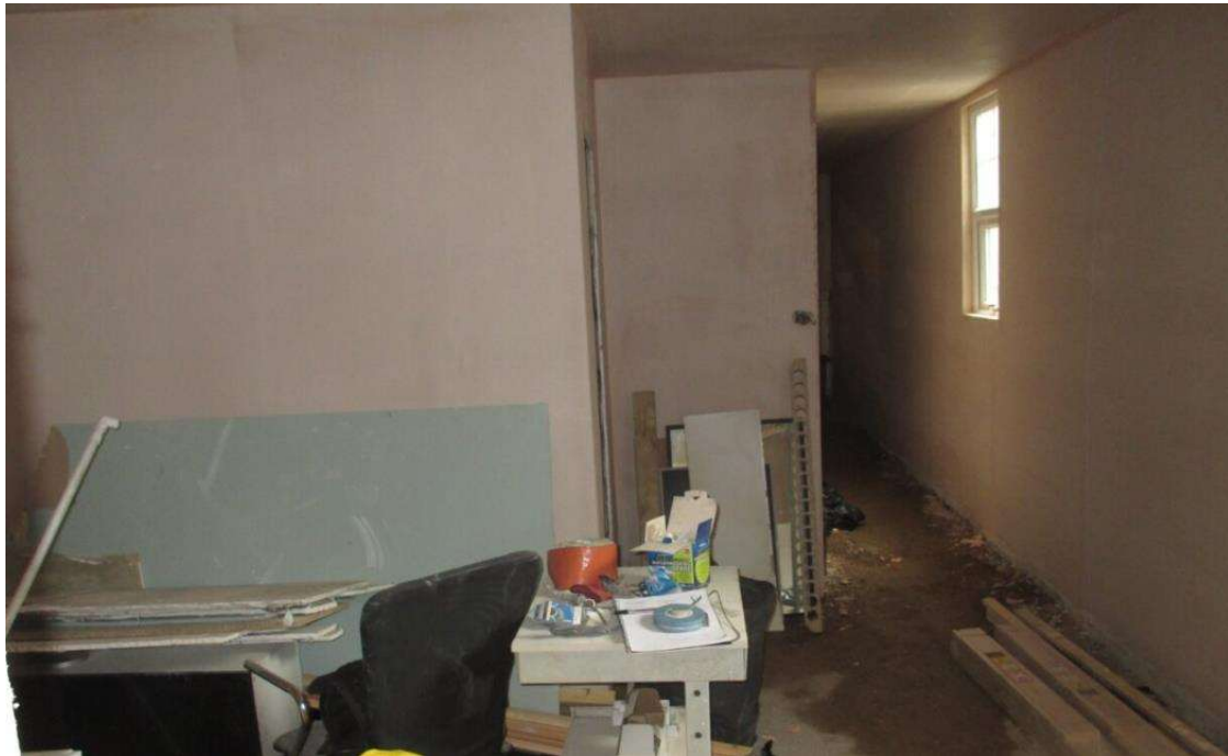
Inside, Internal layout with window looking onto neighbour, out of view a kitchen is being created along with a separate bathroom.
