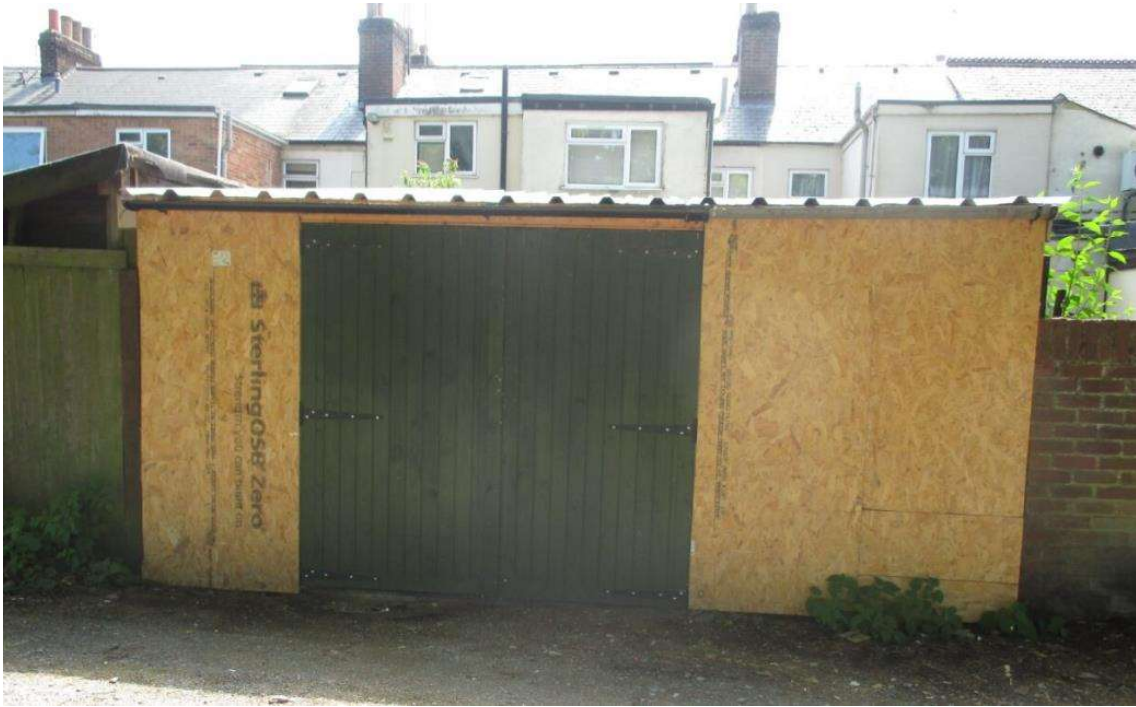
Looking towards the northerly facing (unauthorised) elevation constructed from timber with double timber garage doors.
