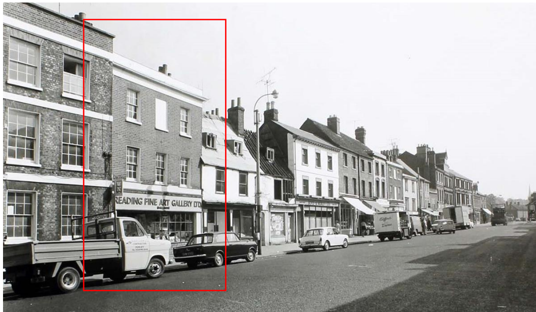
Figure 9: 81 London Street 1971 © Historic England
