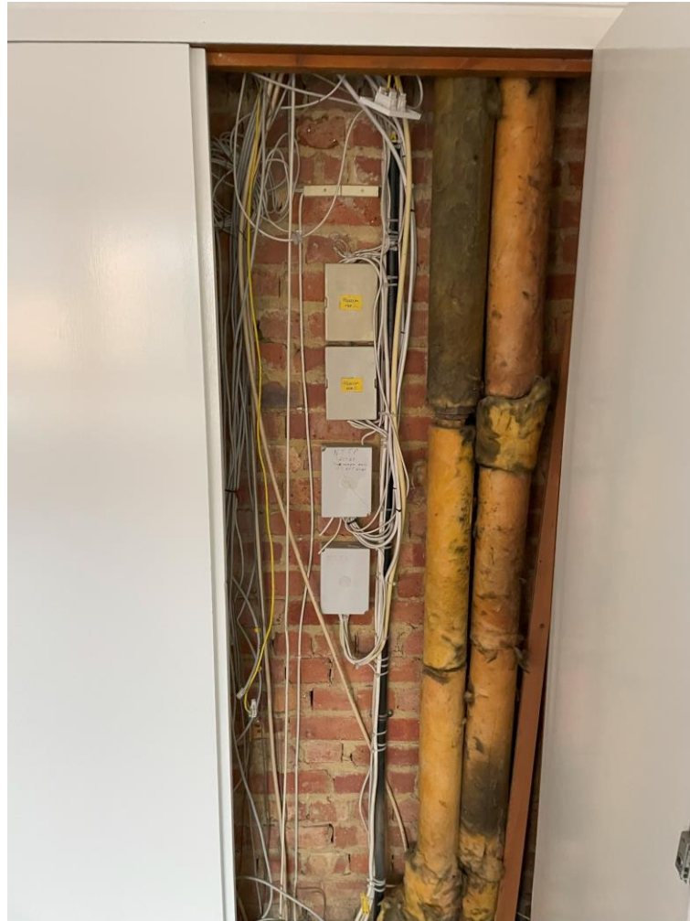
Figure 8: Former rear wall within a cupboard
