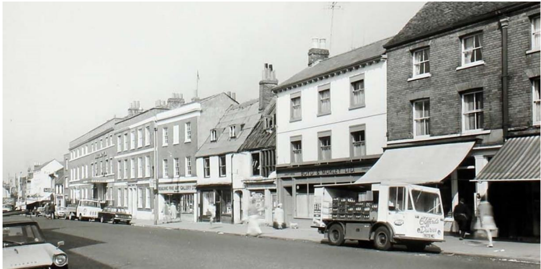
Figure 11: 81 London Street in 1971. The historic roof is still in place. © Historic England
