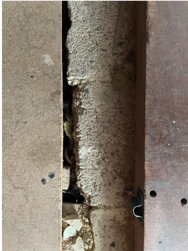
Figure 10: From the loft it is possible to see the materials of the wall below
