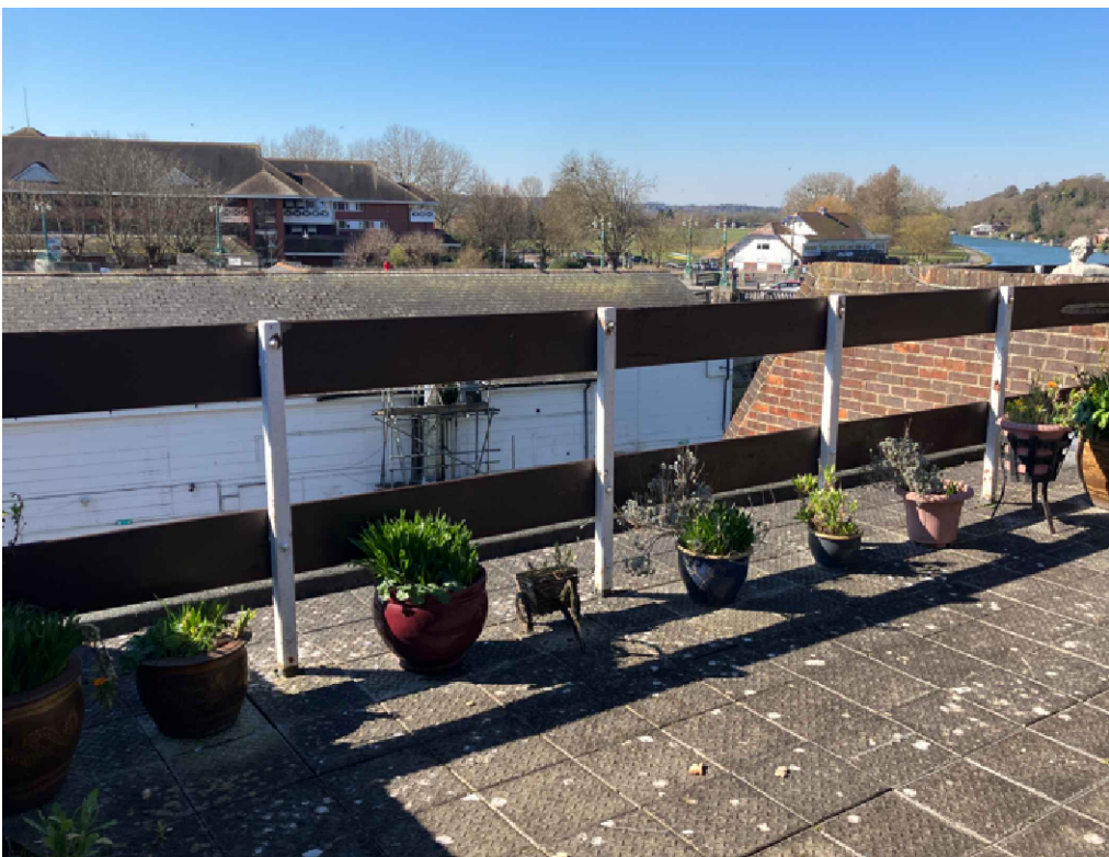
TYPICAL IMAGE OF EXISTING BALUSTRADES
