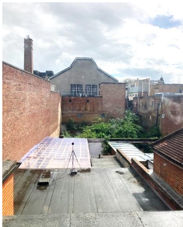
Figure 3 – View facing south, from rear of the existing building
