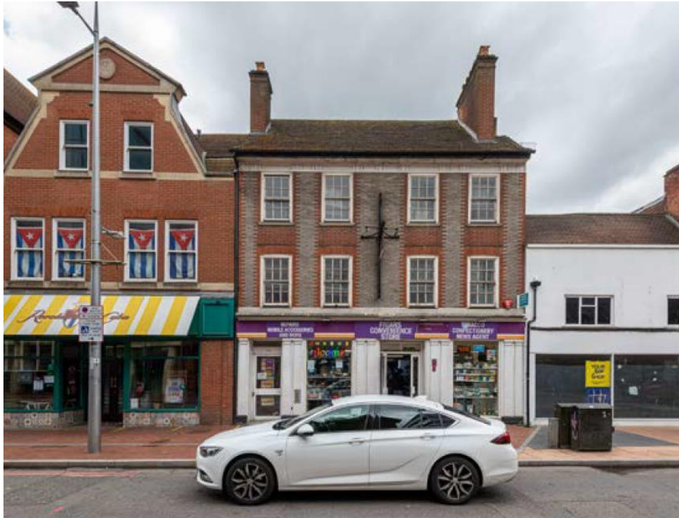
Figure 2 – Street View of the front of the existing building
