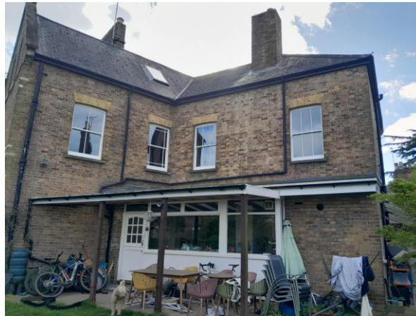
Fig 9: View of the canopy and existing kitchen extension, taken on 30/04/2024
