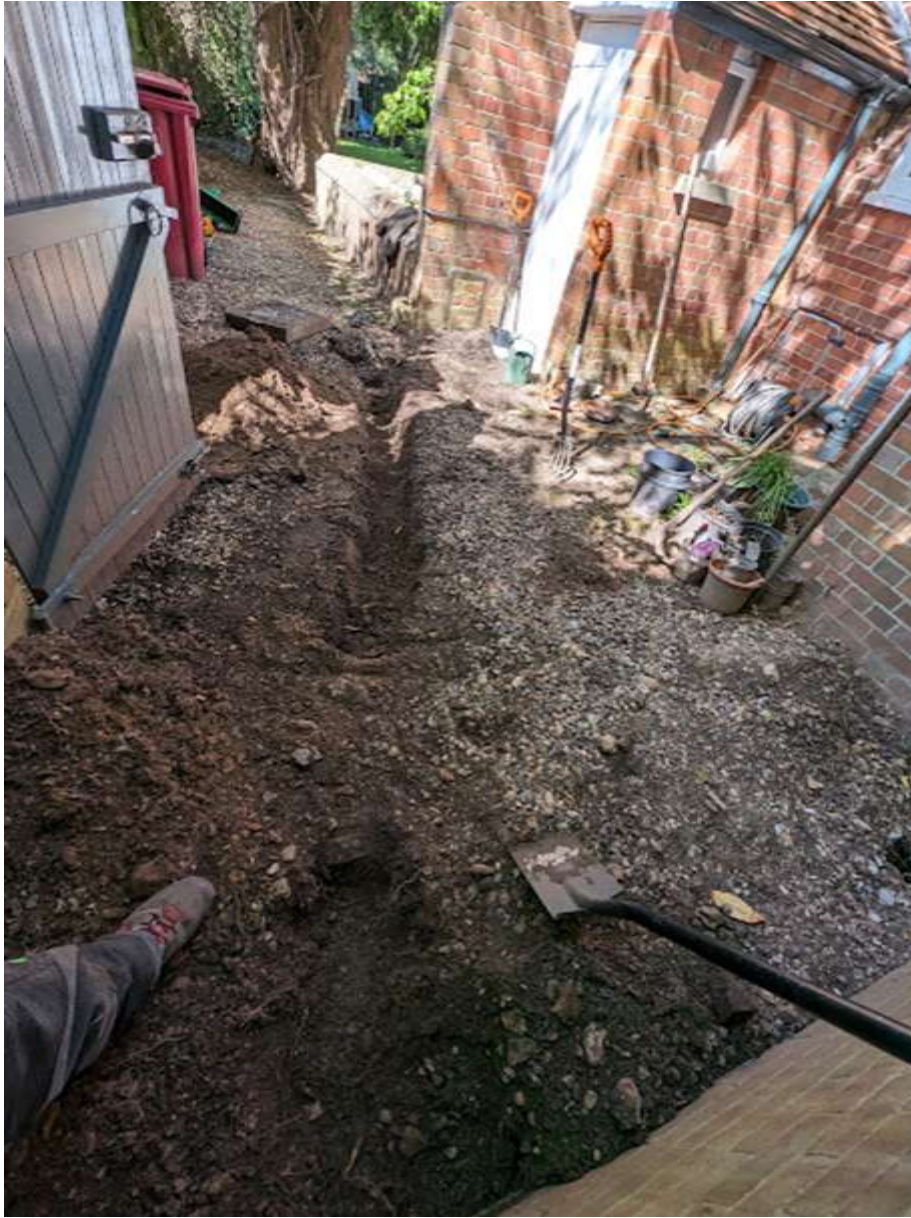
Figure 7: extent of trial pit/trench 2
