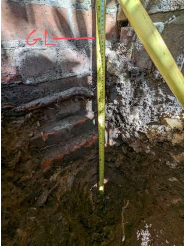
Figure 6: extent of trial pit 1
