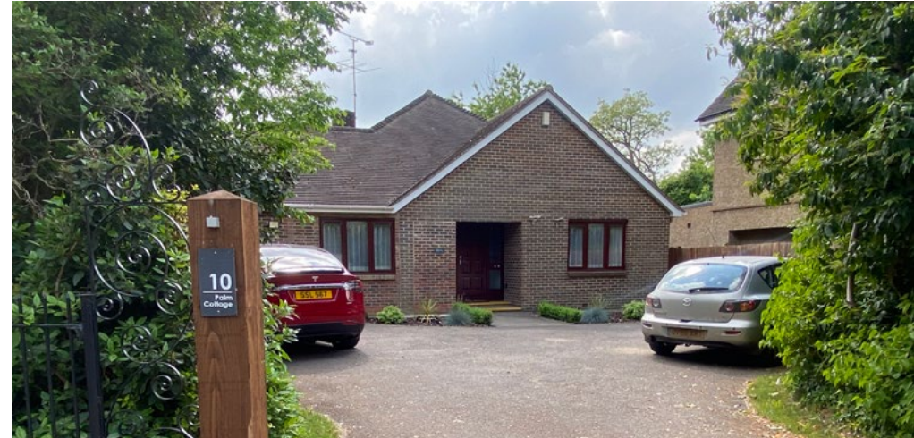
▲ EXISTING BUILDING - front entrance & elevation
