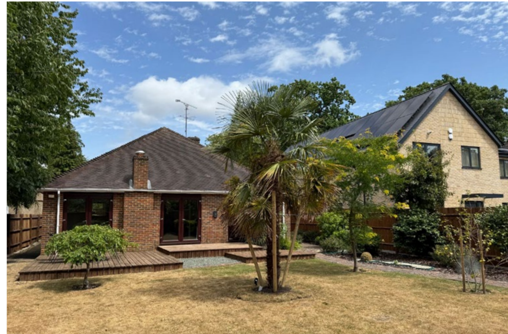
▲ EXISTING BUILDING - rear elevation
