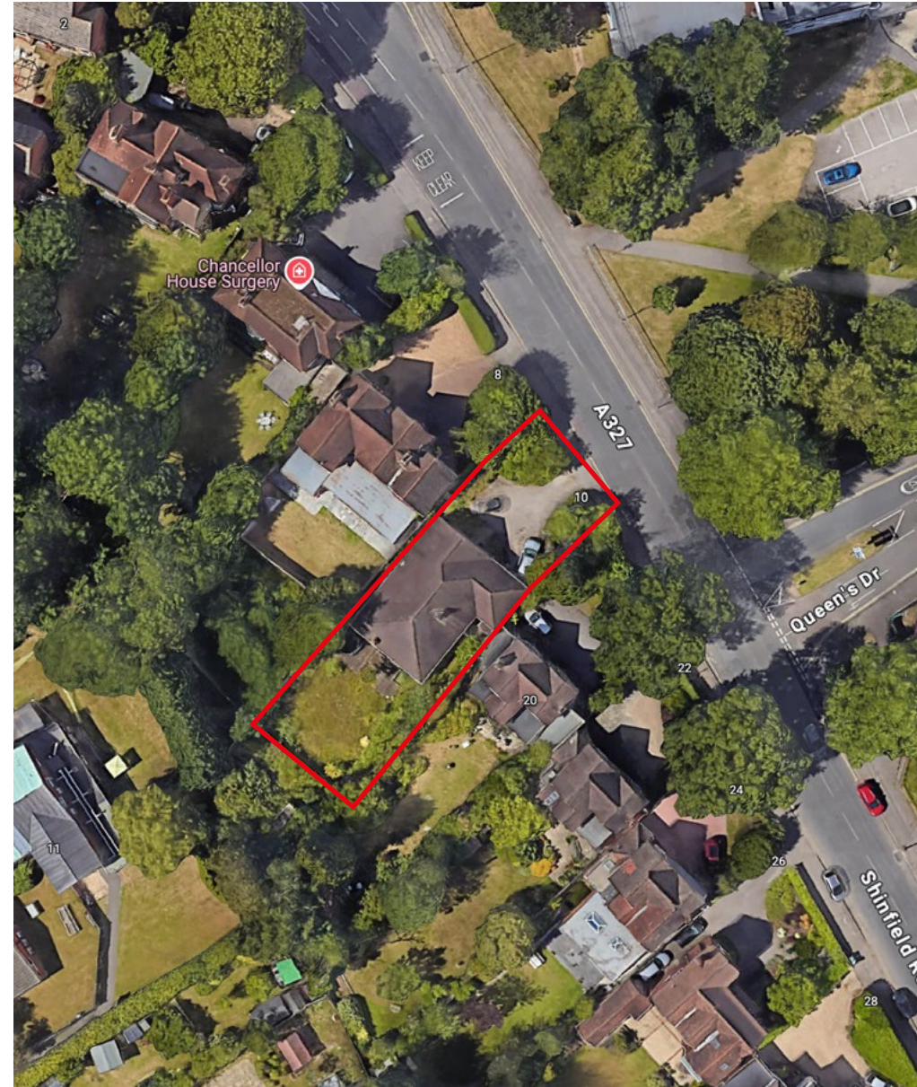
▲ AERIAL IMAGE - the site as existing
