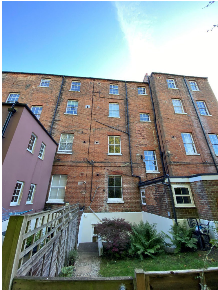
Existing Rear Elevation – View from rear car park
