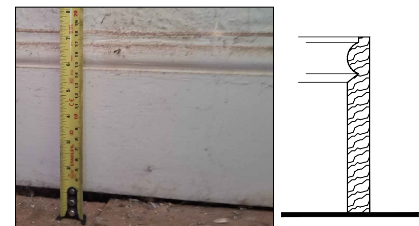
PHOTO: A Proposed timber Torus skirting board to match existing profile and finish
