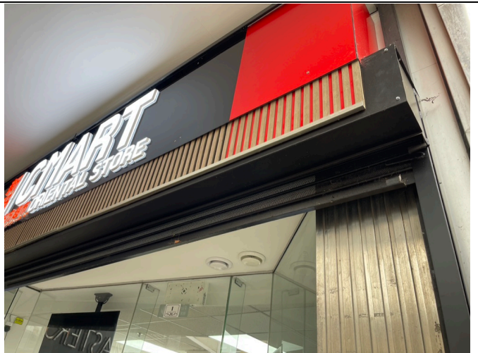
New Signage and roller Shutter Housing Angled Shopfront Glazing and Ramped Threshold
