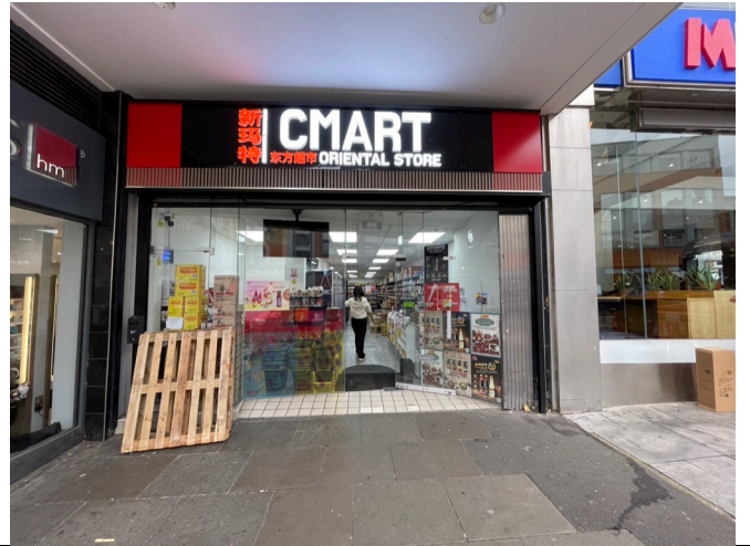
New Signage and roller Shutter Housing Angled Shopfront Glazing and Ramped Threshold
