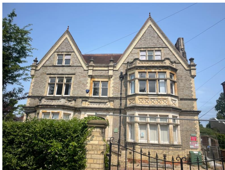
Existing Principal Façade of the building
