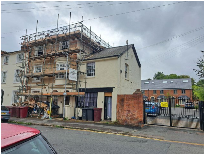
Photo 1 – View of front/side elevation (northwest), 55 and 55A
