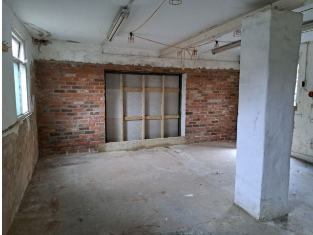
Photo 12 – View of rear extension, ground floor interior, facing south
