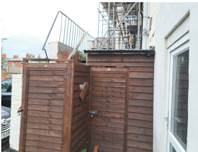
Photo 19 – View of gate leading to stairs to first floor
