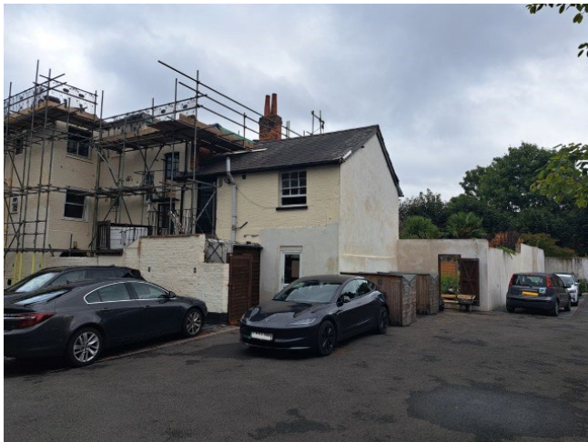
Photo 3-5 – View of rear extension, side elevation (west)
