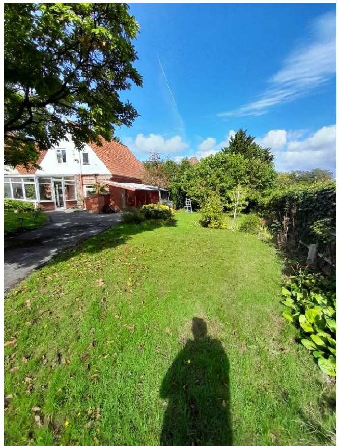
Looking south showing wrap around garden to side
