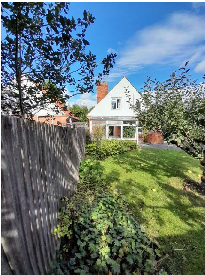
Rear elevation, looking south
