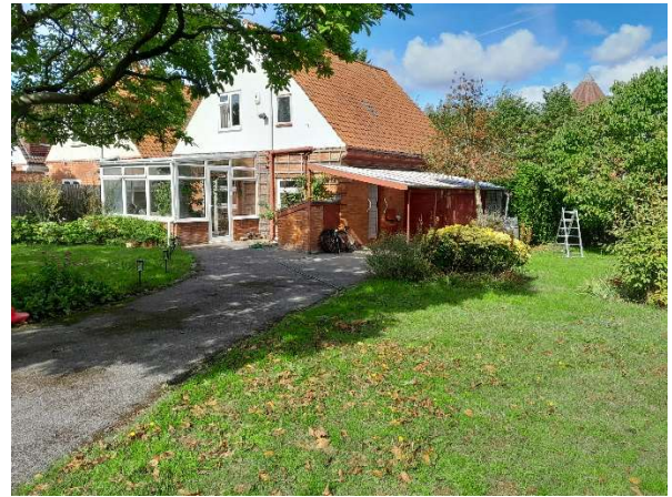
Rear elevation, looking north northwest.
