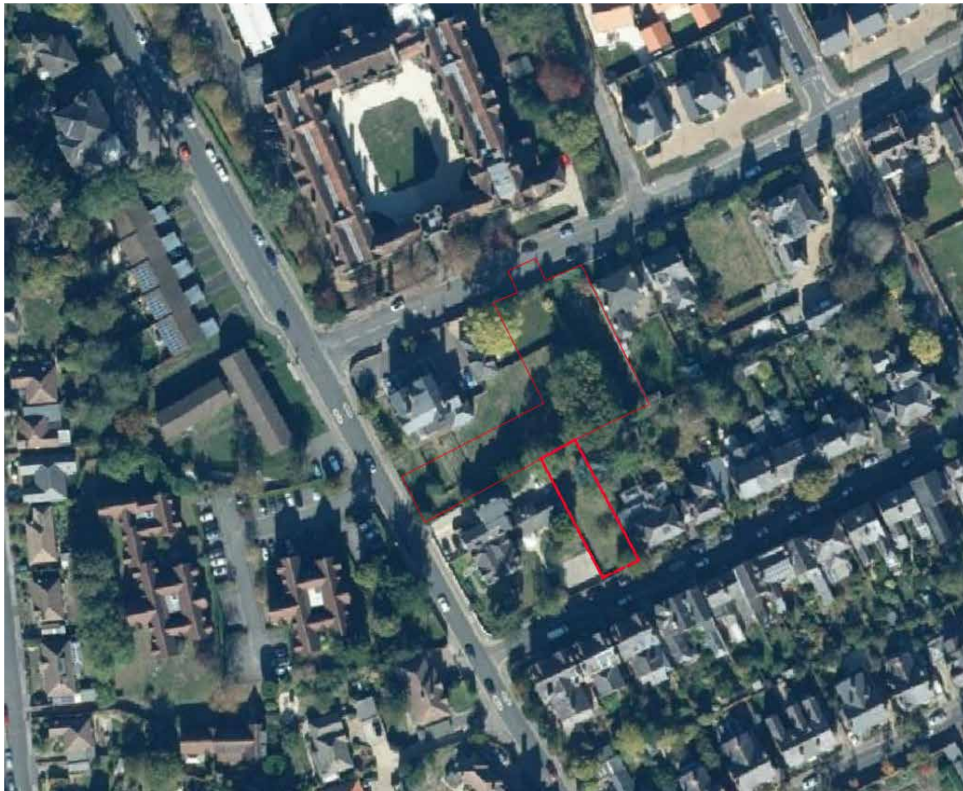
AERIAL VIEW OF THE SITE
