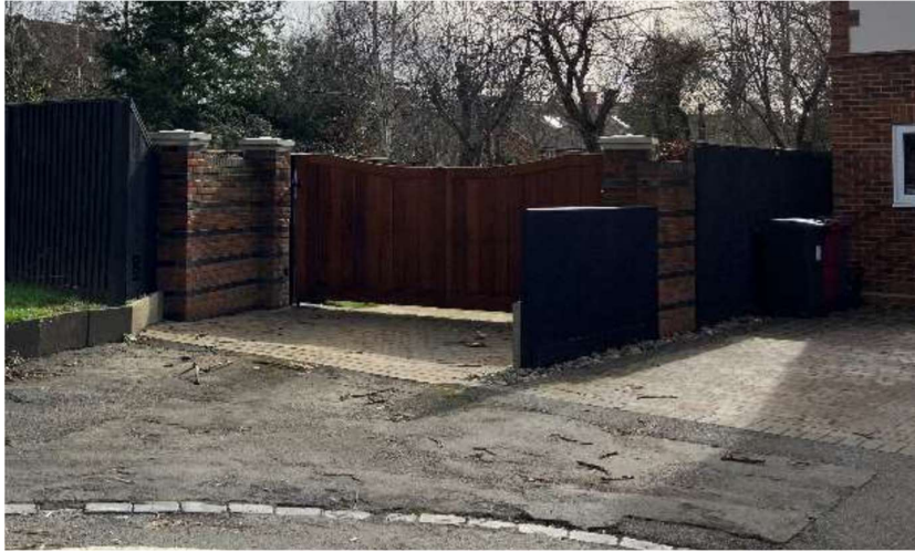
Figure 2 – Photograph of Kearsley Road access
