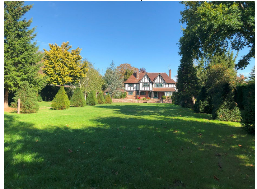
Fig 5. No. 19 Parkside Road showing the rear elevation viewed from the garden.
