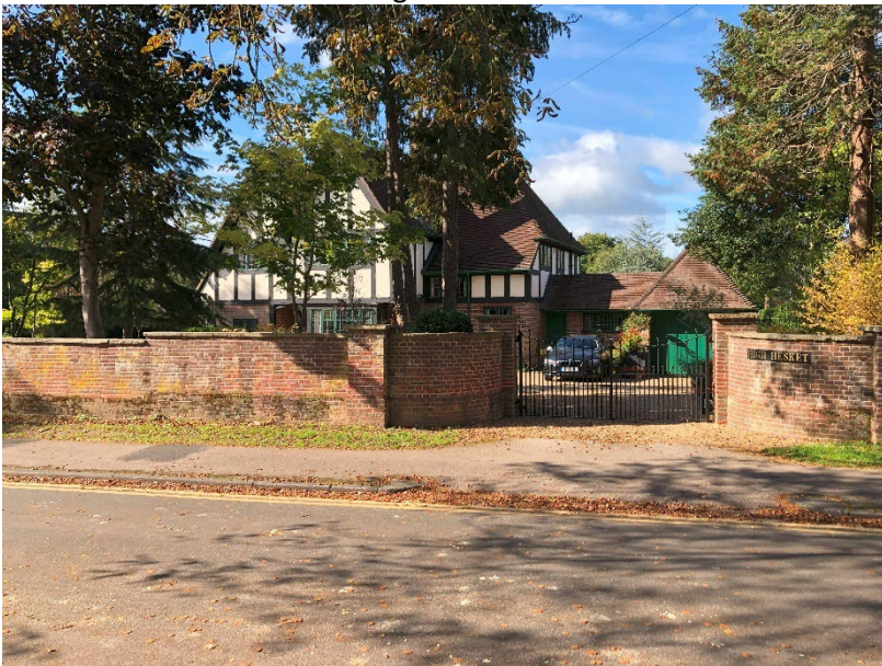
Fig 3. No. 19 Parkside Road showing northern site access.
