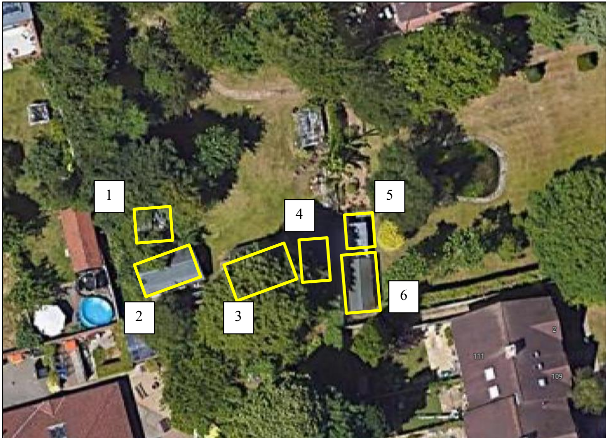
Figure 4. High Heskett building locations; the pond shown to the east of the buildings has been filled in
