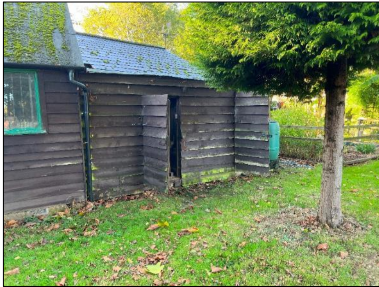
Plate 16. The eastern elevation of building 5.
