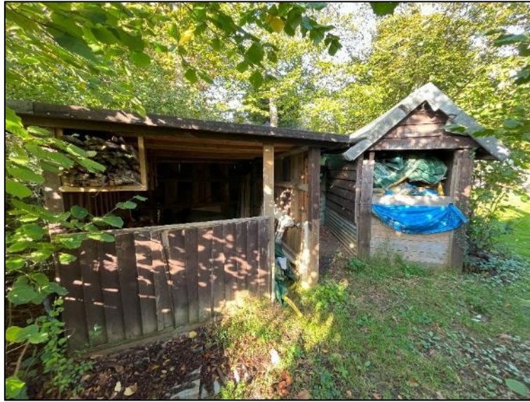
Plate 9. The eastern elevations of buildings 1a and 1b.
