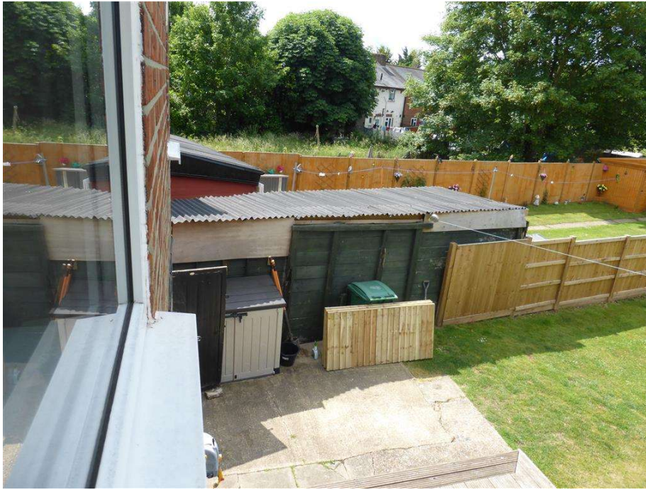
Rear extension and outbuilding 93 Linden Road Reading (now removed)
