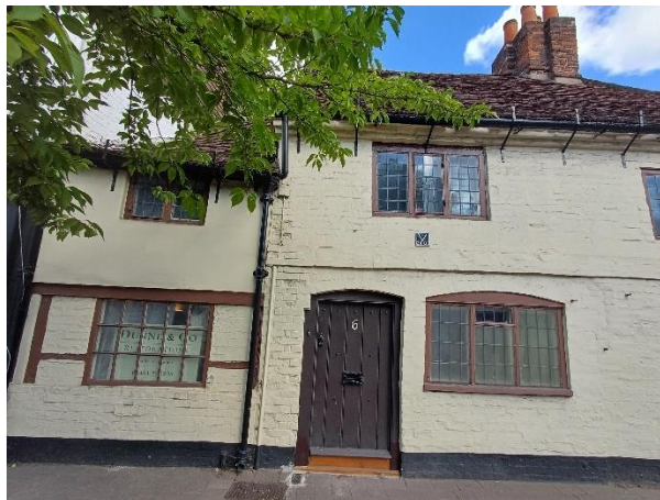
Figure 1: View from the front of 6 Church Street, taken 08/07/2025.
