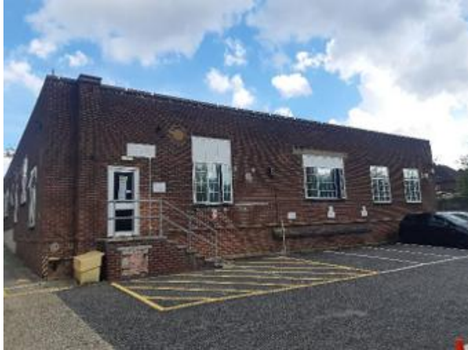
Figure 4. A view of the hard-standing tarmac car park on the western side of the building.
