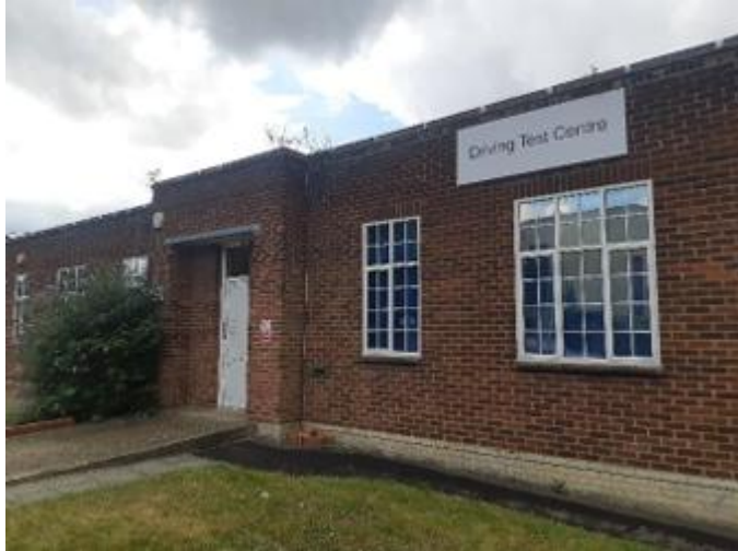
Figure 2. A view of the north-eastern elevation of the building.
