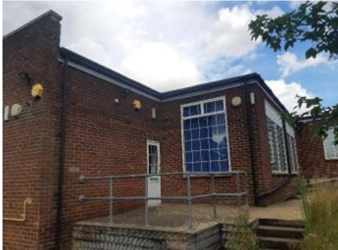
Figure 3. A view of the south-western elevation of the building.
