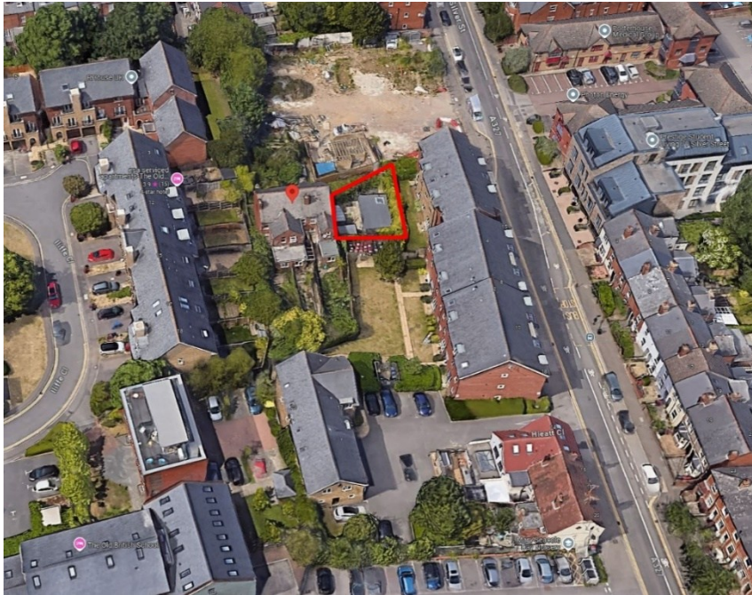
Figure 1: Birdseye View of the Site
