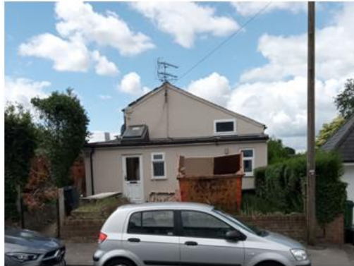
Figure 1 - Adjacent no.37 Chapel Hill
