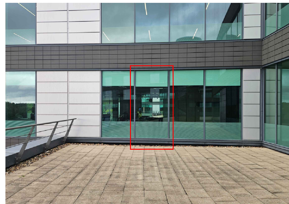
TERRACE DOOR LOCATION
