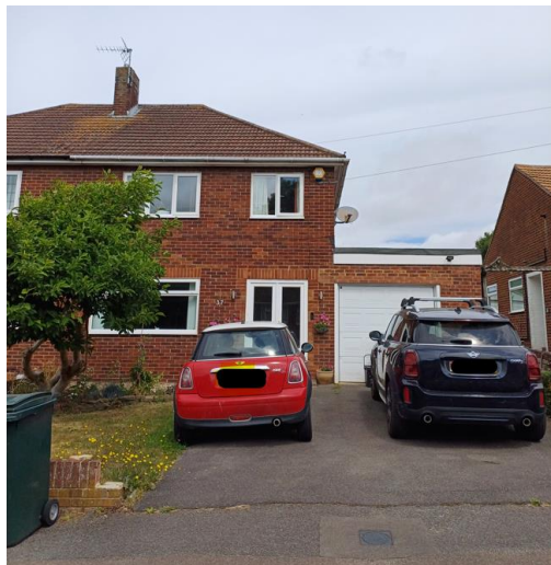
Fig 1: View from the front of the property (24/06/25)
