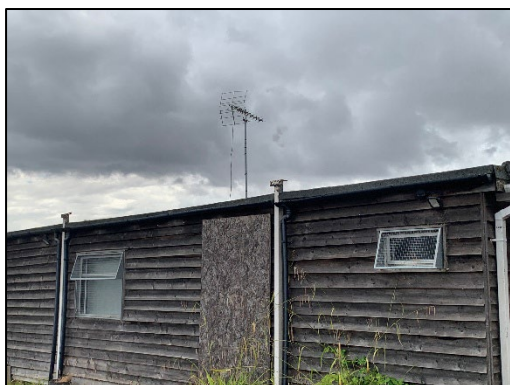
Figure 7: Shiplap extension to west
