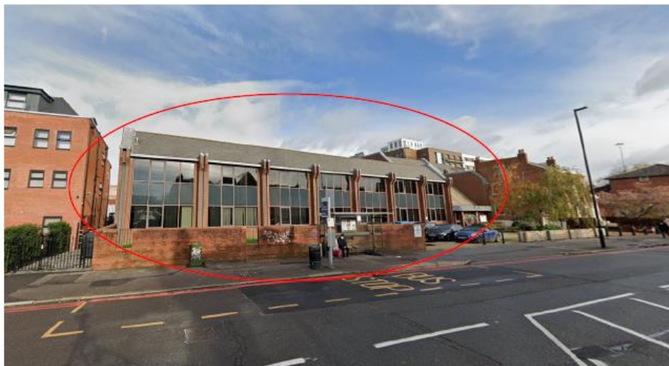
Figure 3: Application building and neighbouring properties – street scene view (Oxford Road)
