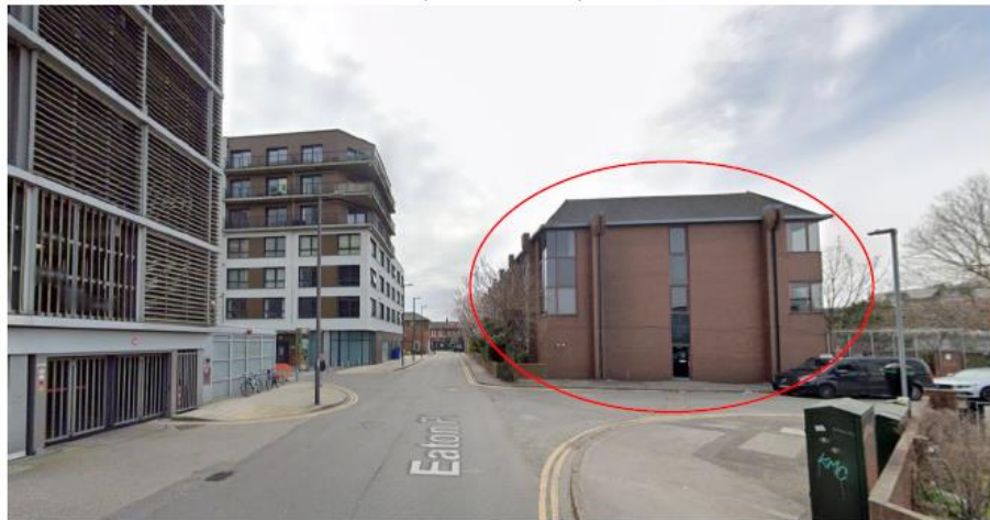
Figure 4: Application building and neighbouring properties – street scene view (Eaton Place towards Oxford Road)
