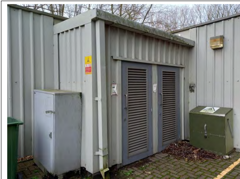
Photo 11: Disused gas house
