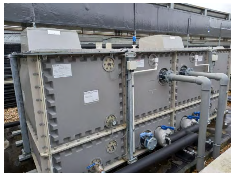
Photo 2: One of the two water tanks at roof level
