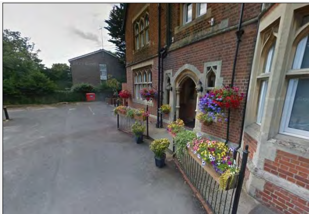
Plate 7: From southeast of property facing west across car park showing front entrance and hardstanding car park
