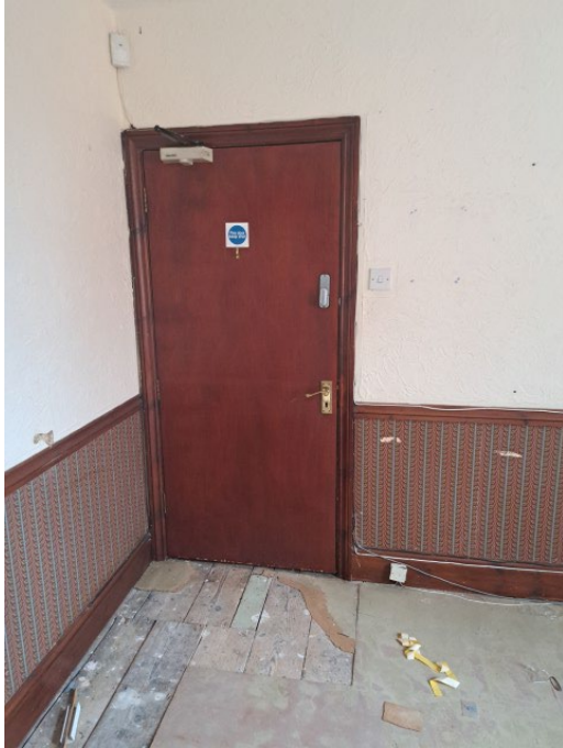
Photo 15 – View of doorway to first floor rear room
