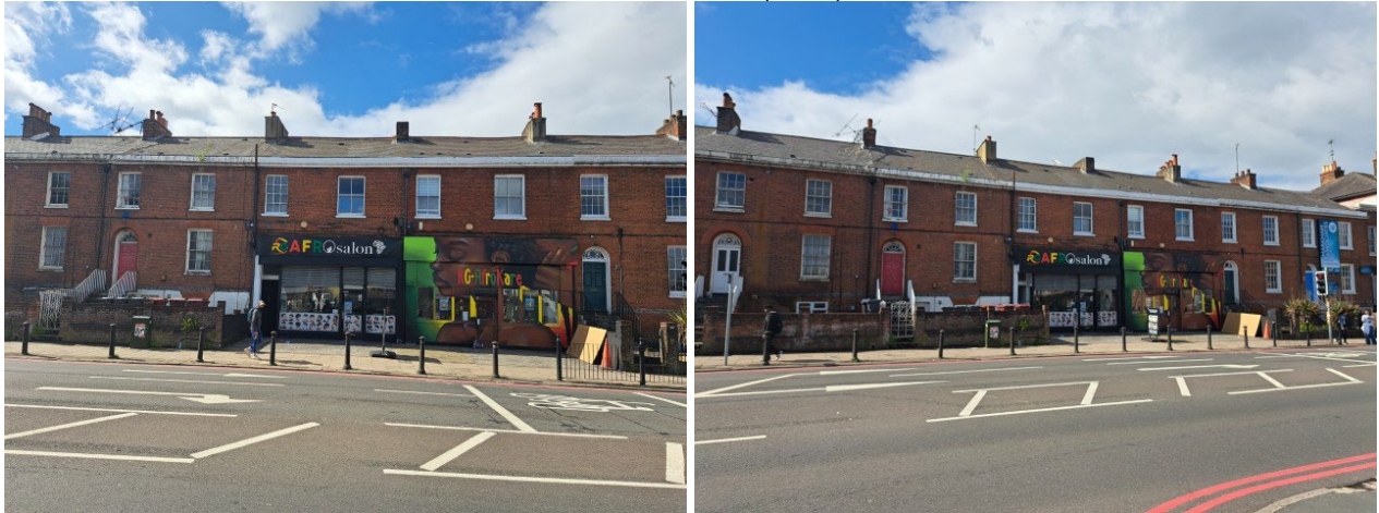
Photo 1 – View of front elevation (north)
