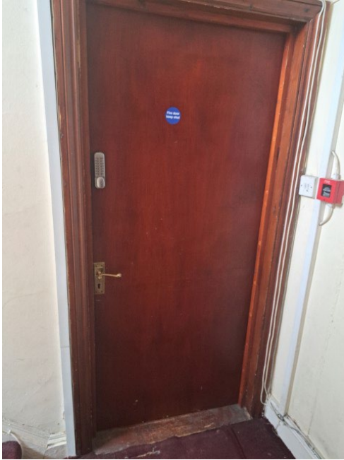
Photo 8 – View of entrance to first floor space
