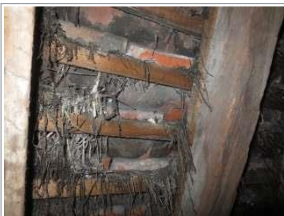
Roof tiles loft
