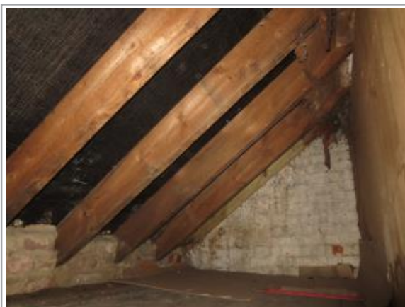
Bed 3 eaves void
