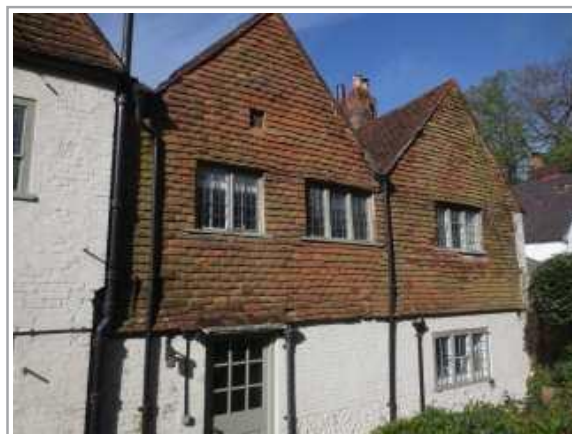
Tile hung walls rear
