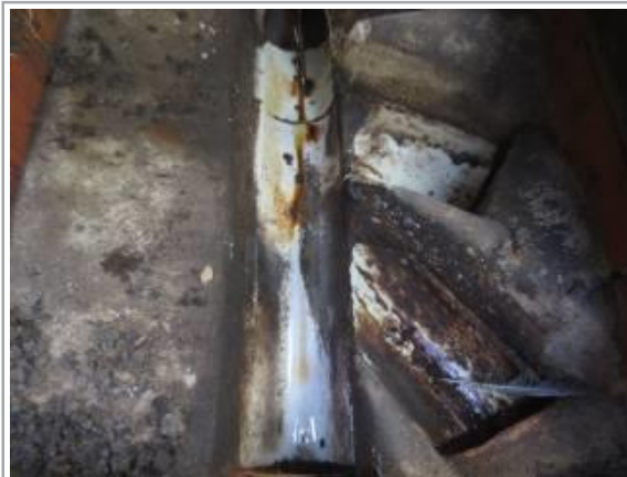
Shallow drains rear.
