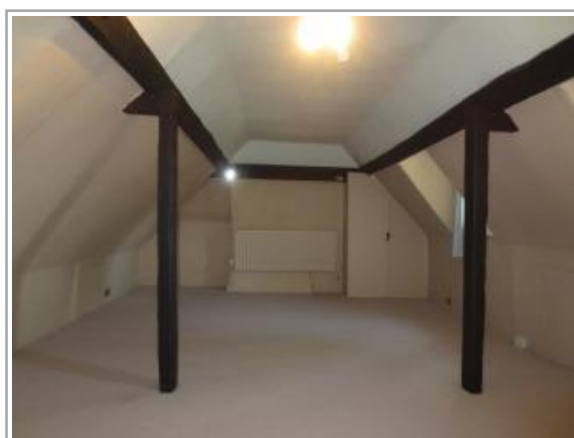
Bed 2 roof frame
