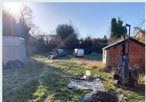
A view of WS04 towards the Southwest
