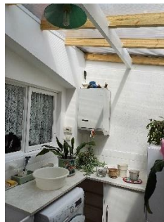
Site visit - Location of the boiler that needs to be replaced
