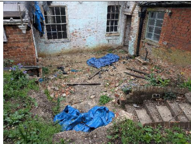
Picture 4: Partially removed hardstanding to the west of B1
