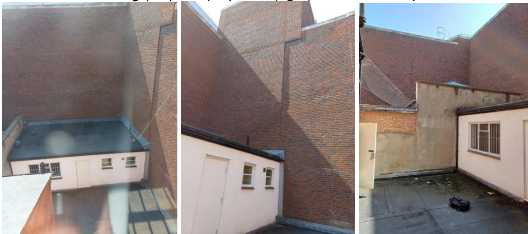
Site photographs from third floor (left) and looking west (middle) and east (right)
