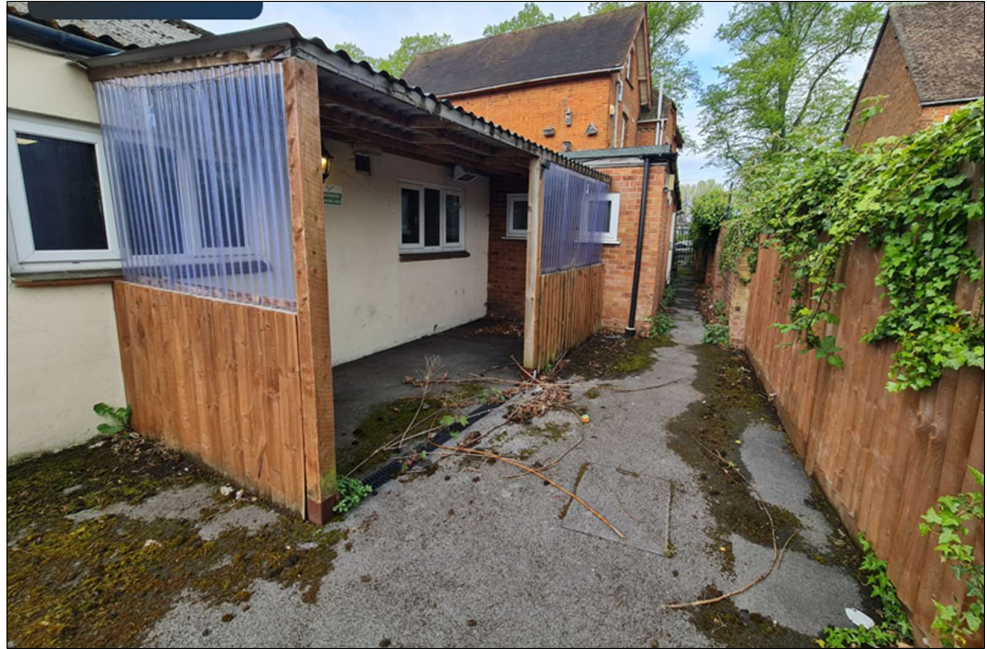
Figure 4: Photograph of rear extension
