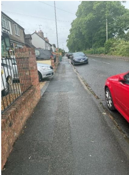
Photograph 3: Pedestrian Footways on Kentwood Hill (eastern side of carriageway)
