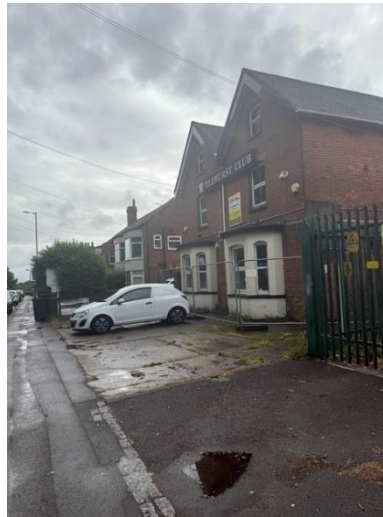
Photograph 1: Existing conditions of the site
