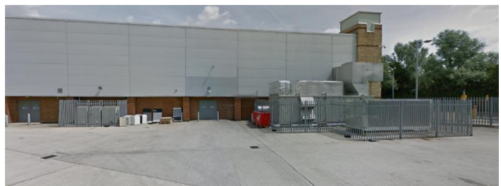
Image of compound at rear of Unit 5 Curry's
