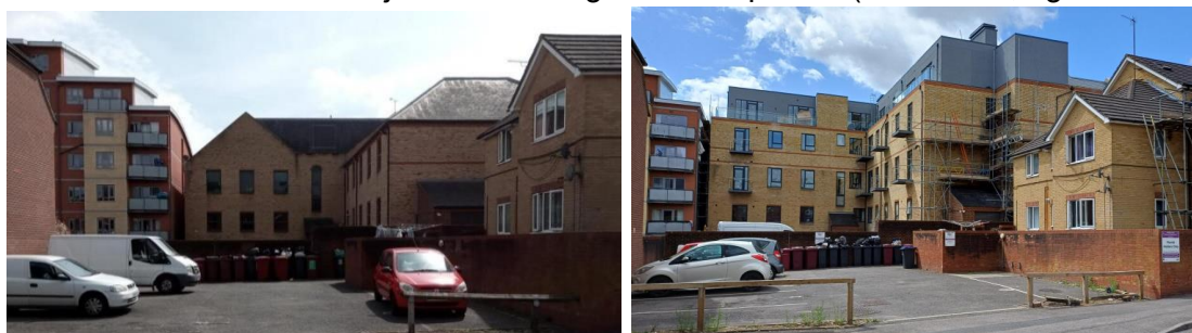
The rear of the site, from Norwood Road, looking south (left: 9/5/2022; right 5/8/25).
