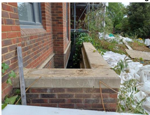
Photos showing the raised surround of the lightwell (left) & basement level (right).
