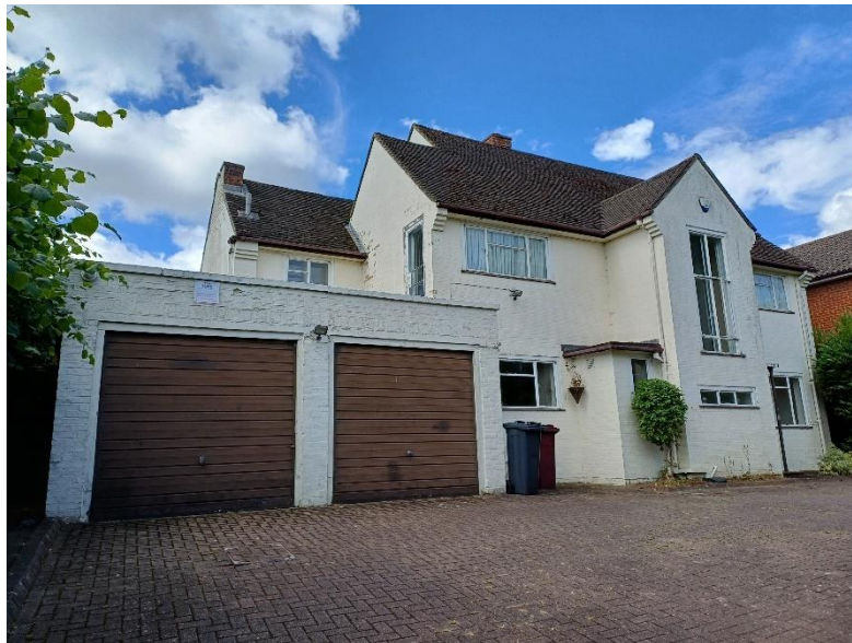
Fig 1: View from the front of the property, taken 07/07/25;
