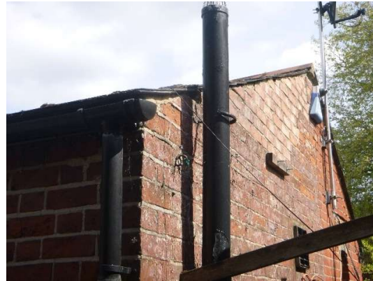
Photograph 8. Verge mortar on gable mostly intact (rear elevation).
