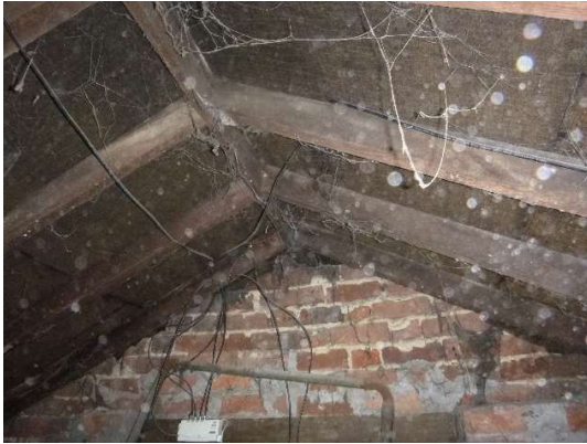
Photograph 14. Bitumen roof felting and heavily cobwebbed ridge (loft space).
