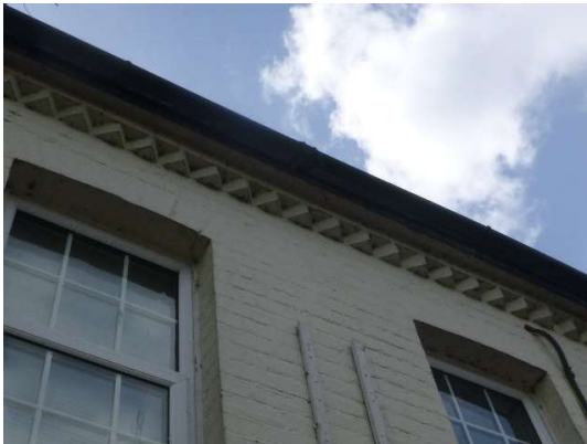
Photograph 13. Ornate brickwork at eaves (front elevation).
