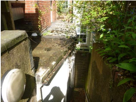
Photograph 5. Stairs leading to ground floor of property (u~829).
