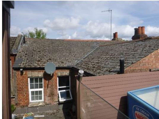
Photograph 2. Rear of property viewed from poolside bar area to south (u1b5).
