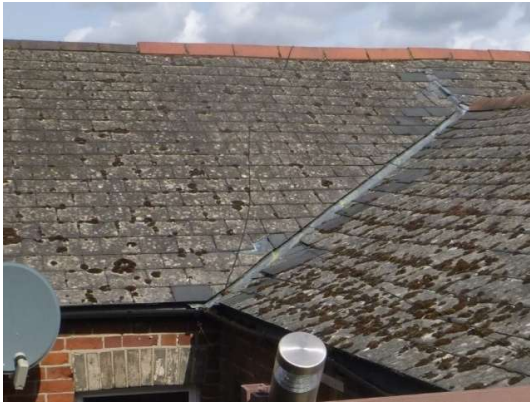
Photograph 7. Flat, intact slate roof tiles (rear elevation).
