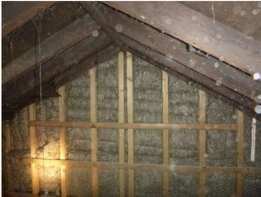
Photograph 16. Eastern party wall (loft space).
