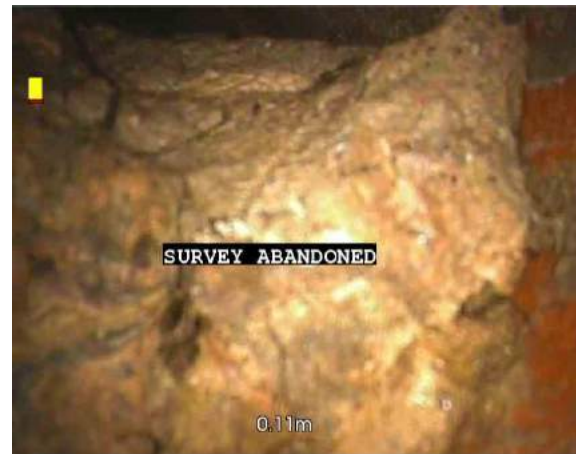
2, 00:00:13, 0.11 m Survey abandoned, Unable to pass due to silt deposits
