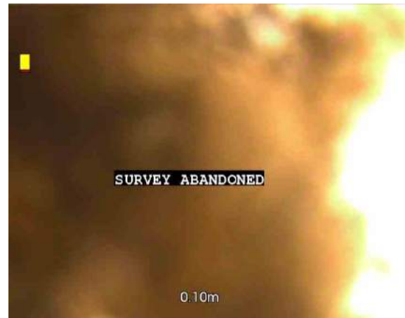
2, 00:00:19, 0.10 m Survey abandoned, Unable to pass due to silt deposits
