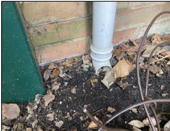
RWP 7 - ONTO GROUND
