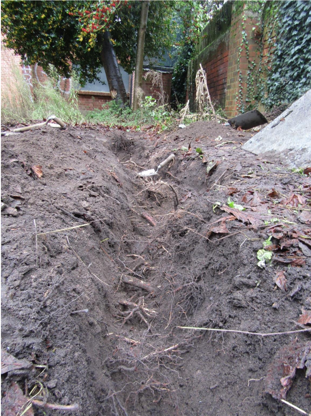
Completed trench with exposed roots.
