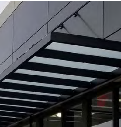
PROPRIETARY GLASS CANOPY ABOVE ENTRANCE DOORS
