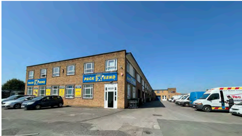
12: EXISTING EMPLOYMENT BUILDING ALONG MILFORD ROAD
